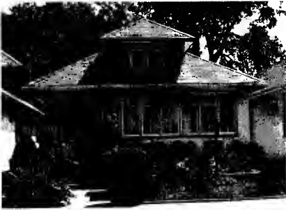
Figure 1: 7641 South Merrill Avenue
